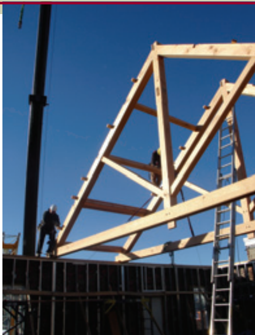
First two trusses are tied together with 8-inch by 8-inch purlins.
